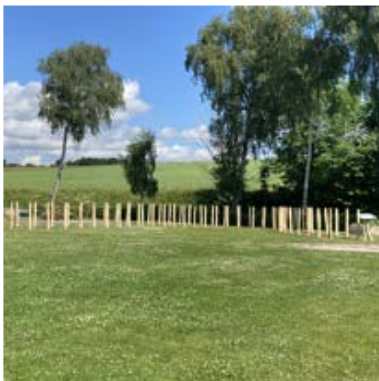
Figure 7. Brush fences before (left) and after (right) filled with branches and garden waste at the Knudsøskolen (elementary school). The width is typically 1,5 meter and height 1,2–1,7 meter. The poles are embedded 1 meter in the ground for the stability of the filled fence (Photos: renosyd).
